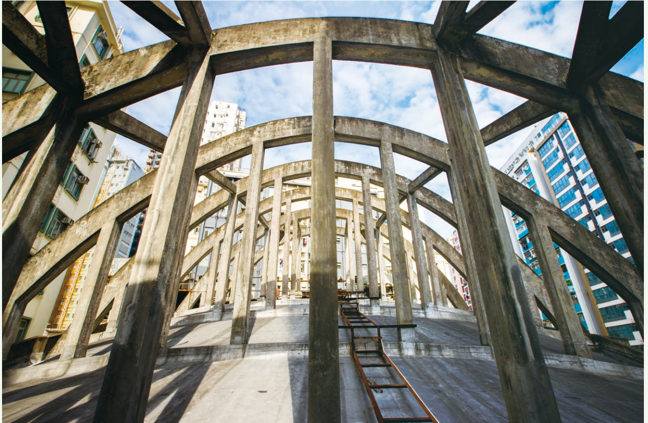
The iconic parabolic exoskeleton truss of State Theatre
